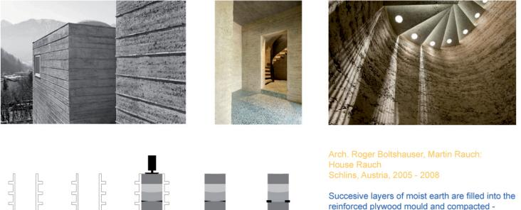
ideal mixture of earth: 15-18% clay 23%coarse aggregate 30% sand 32% silt mortar layers, stone slabs, metal or fired strips of ceramics can be applied as erosion brakes
