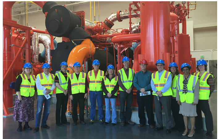
Stanford's new energy system is reducing GHG by 68% and saving $420 million over 35 years. Photo credit: Stanford University
