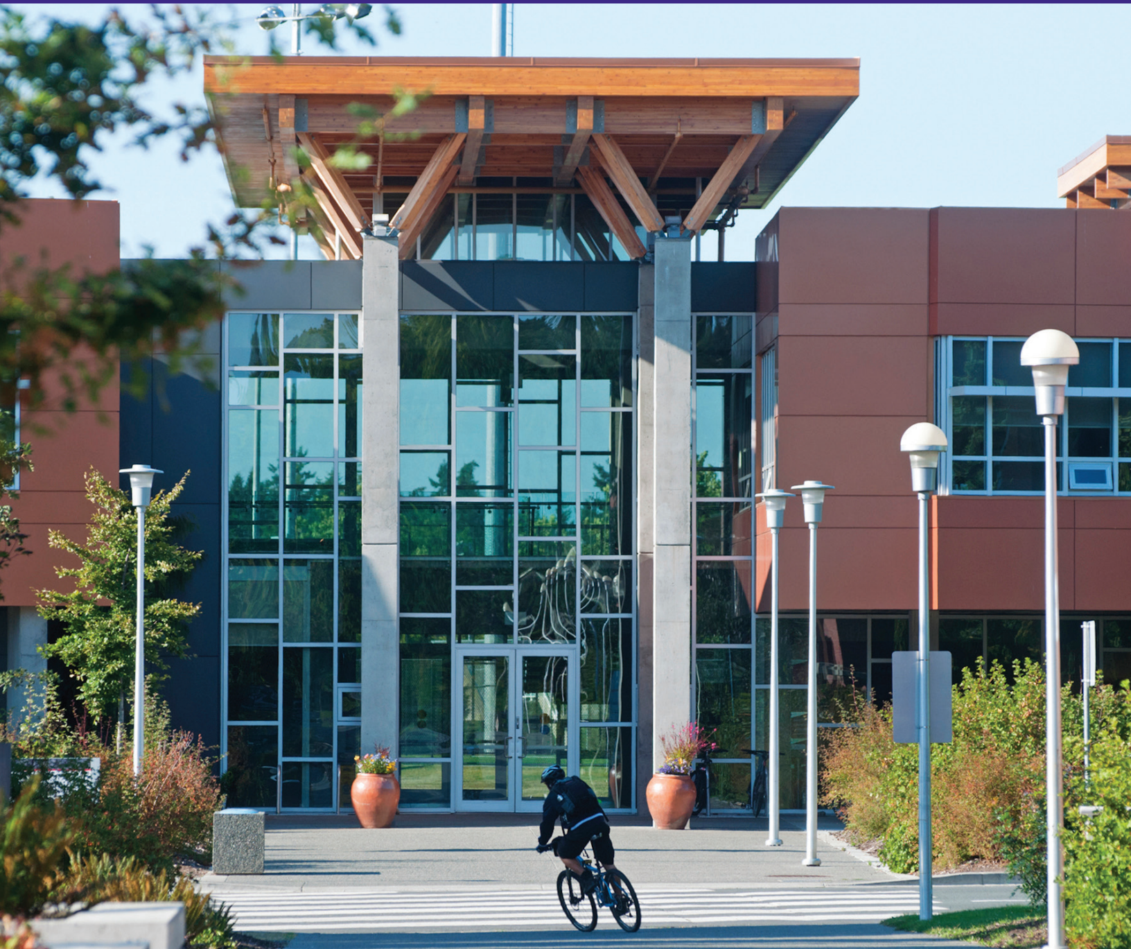
University of Victoria's LEED Gold Administrative Services Building. Photo credit: University of Victoria
