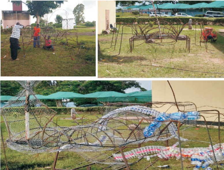
Figure 5. Construction of the main frame of the scorpion model disposal basket.
